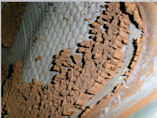
Potable Water Treatment
